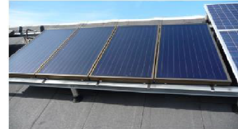
Figure 33. Module of 4 flat plate collectors of the solar heating system.
